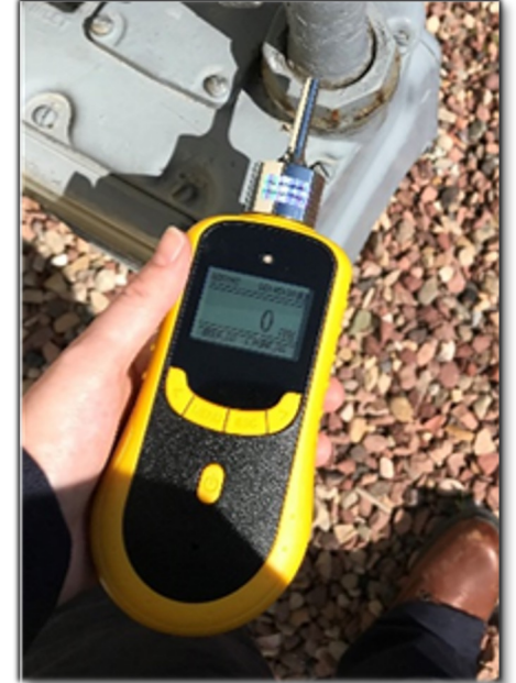
Testing for hydrogen leaks.
